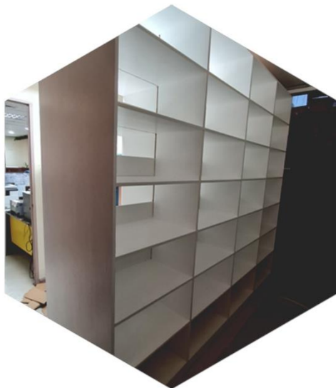
Fabrication & Installation of Shelves in COA File Room @ 8th floor MAB
