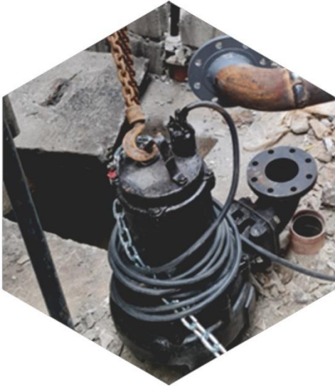
Installation of Submersible Pump at Annex Building Septic Vault
